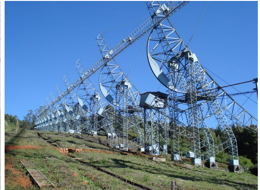
The Ootacamund (Ooty) off-axis parabolic cylinder 530 m long and 30 m wide (15,900 m 2 ) operating at a nominal frequency of 326.5 MHz
