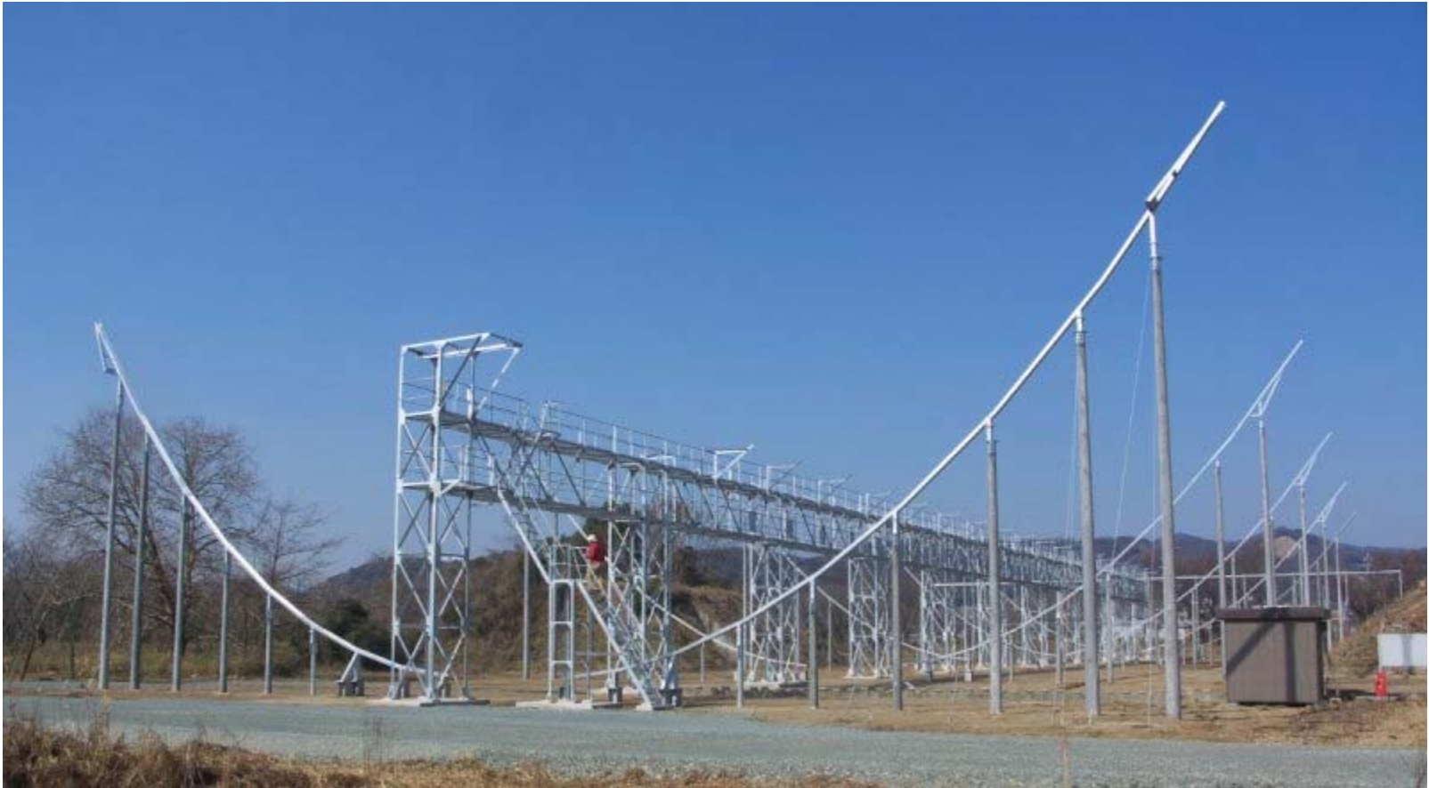
New STELab IPS array at Toyokawa - photo February 17, 2007 (array now operates)
