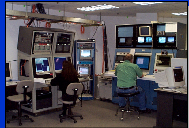
Observatory Control System
